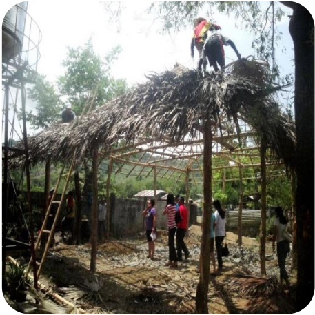
Installation of labig roofing
