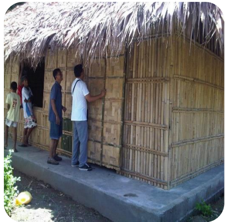
Installation of sliding bamboo door
