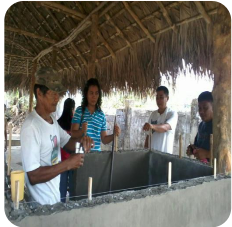
Installation of CHB wall for the toilet using bamboo for
