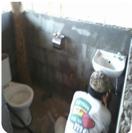
Installation of plumbing fixtures
