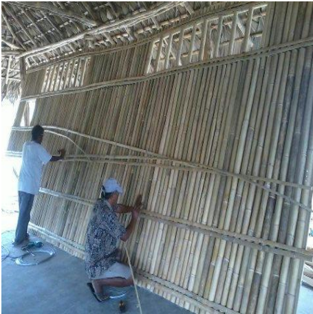
Construction of bolo walls
