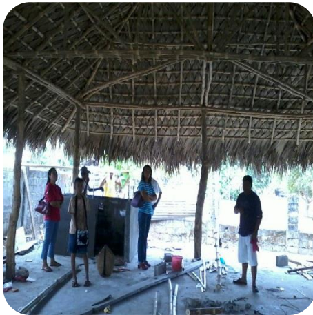
Completed labig roofing
