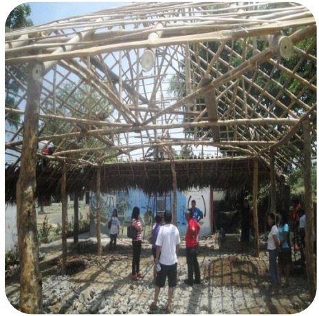
Installed kakawate posts and bamboo trusses
